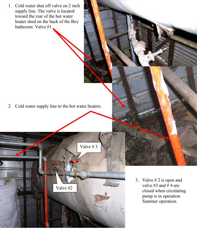
4. Valve # 2 and # 4 are closed and valve # 3 is open when circulation pump is not in operation. Winter operation.
