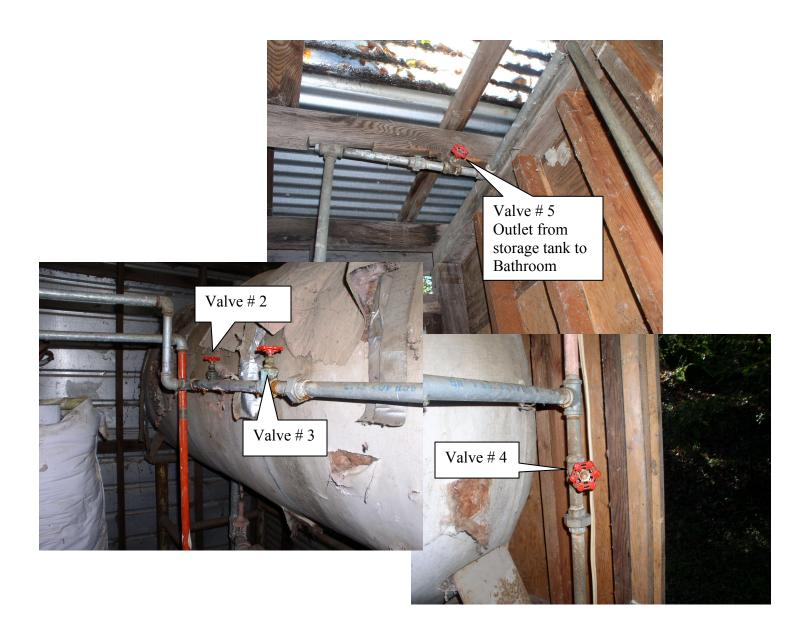
6. Valve # 5 should be closed when circulating pump is not in operation, Winter operation
